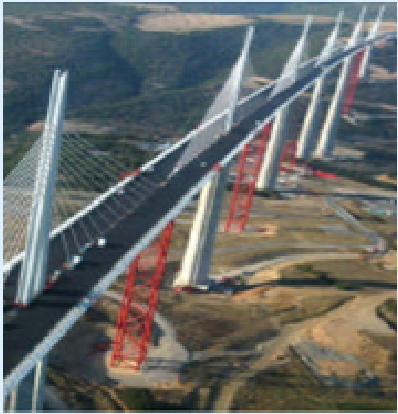
Viaduct de Milleau over 21,000 t plate from Dillinger Hütte
