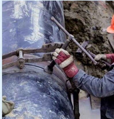
Gas pipeline project 1420 mm
